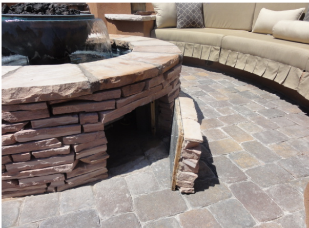
Stone enclosure on site
